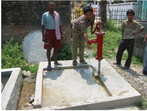
Water supply well completed by LEI workers in Dhanusha, Nepal
